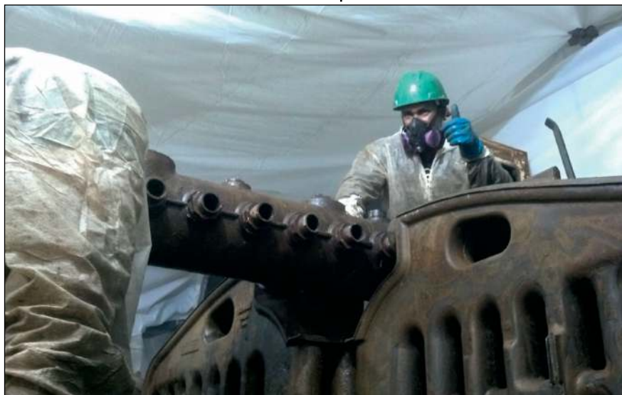
A worker deals with abatement and demolition of a boiler with asbestos at a high school.
